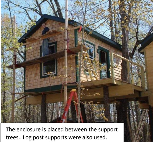
The enclosure is placed between the support trees. Log post supports were also used.
