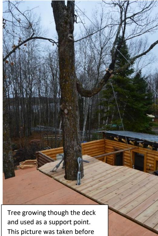
Tree growing through the deck and used as a support point. This picture was taken before the walls were erected.
